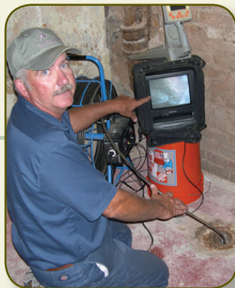
Ken Wilkerson points to the monitor showing an example of a good section in the CFT sewer line.
